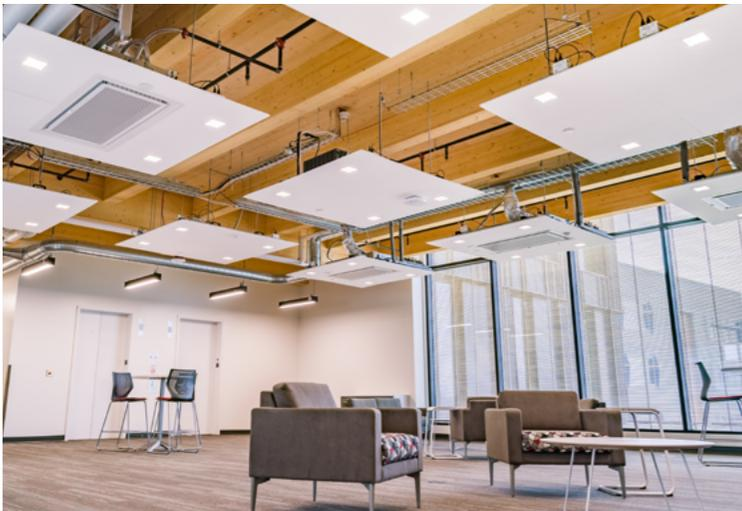
The **Catalyst building**, in Spokane, Wash., employs pioneering efforts, such as cross-laminated timber, daylighting and air sealing, to hit zero-energy and zero-carbon targets. The design of the building ensures that the building remains functional without power.
